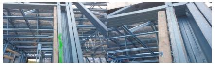
• Bow in corner of opening Hallway / rear Garage door. Corner stud variation exceeds 4 mm in 2 meter building tolerance standard
