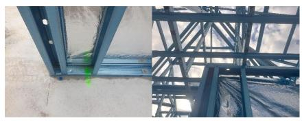
Install anchor bolt in bottom plate directly adjacent stud right side of Study opening to maintain tie down as tie down point of gable roof truss directly above.
