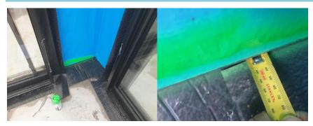
Frame on right side of Hallway sliding door overhangs slab in excess of tolerances requirement 15 mm maximum for 90mm frame overhangs slab by 17 mm to 25 mm in corner.
