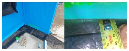
Frame on left side of Dining Room sliding door overhangs slab in excess of tolerances requirement 15 mm maximum for 90mm frame overhang slab by 20mm in corner.
