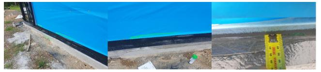
Frame on Main Bedroom external wall section overhangs slab in excess of tolerances requirement 15 mm maximum for 90mm frame overhang slab by 20mm mm in corner QBCC Standards & Tolerances Standard Section 5.11
