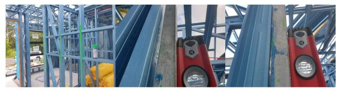
Corner to middle of Hallway / Bedroom 4 robe wall out of plumb exceeds building tolerance 4 mm in 2 meters
