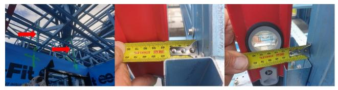
2 Gable roof trusses above Study window adjacent Master Bedroom 30mm out of plumb exceeds building tolerances requirement / rectify
