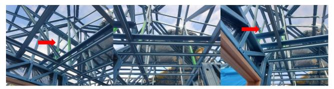
• Gable roof trusses, 3 over front Study / Bedroom 4 walk-in robe out of plumb
