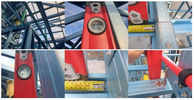
Gable trusses over front study, Bedroom 4 & Walk in robe leaning out of plumb between 20mm and 40 mm
