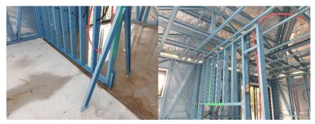
Wall frame between Master Bedroom and Ensuite recess in wall top head bowed down and areas of damage to top plate not tied to ceiling diaphragm. Base of wall unsupported.
