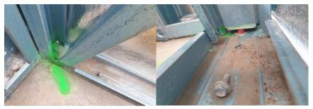
Gap under cyclone washer incorrectly installed on anchor bolt bracing panel rear left corner of Bedroom 4 sliding door opening
