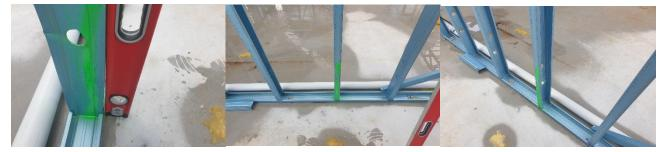
• Stud base damaged on Hallway / Garage wall damaged requires repair / bow in base of stud
