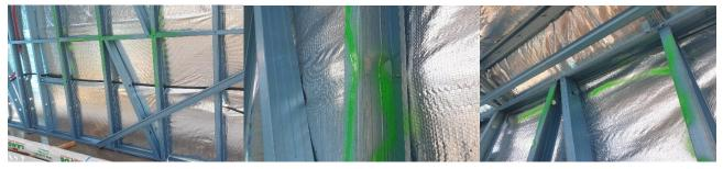
Various splits and damage to wall plates, studs & noggings garage side wall
