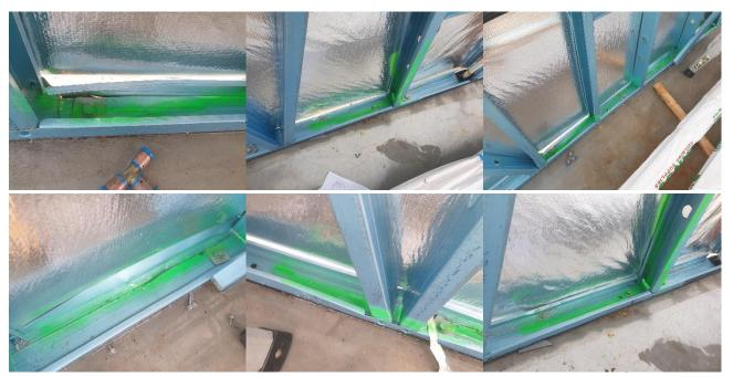
• Damaged garage wall framing top / bottom plates wall out of plumb. Splits in framing right side garage wall. Due to the extent of damage to top, bottom plates, studs and noggings wall would need to be replaced. Damaged structural component splits in metal frame.
