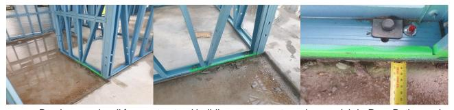
Bracing panel wall frame structural building component overhangs slab in Rear Bathroom by 20 mm. Slab edge support / repair for frame with structural grout required.
