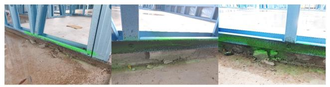
Anchor bolts on ends of bracing panel slab edge Rear Bathroom damaged. Slab edge / anchor point requires rectification to meet structural building requirement.
