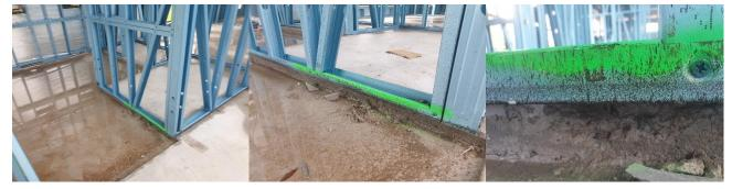
Main Bedroom Ensuite damage to slab edge where anchor bolt installed on bracing panel side wall adjacent opening from master bedroom. Wall frame bracing structural component overhangs slab edge by 30mm exceeds building tolerance. Wall frame slab edge should be supported with high strength grout / structural bracing component.
