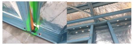
Stud front right side of garage wall direct support under roof truss above cut out and not correctly attached to bottom wall frame additional stud should be placed directly beside
