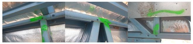
• Multiple kinks and damage to wall framing and face plate on left side of garage door head
