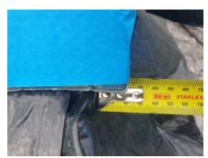
External wall frame on left rear corner of Main Bedroom Ensuite overhangs slab edge in excess of tolerances requirement 15 mm maximum for 90mm frame overhangs slab by 20mm exceeds QBCC Standards & Tolerances Standard Section 5.11
